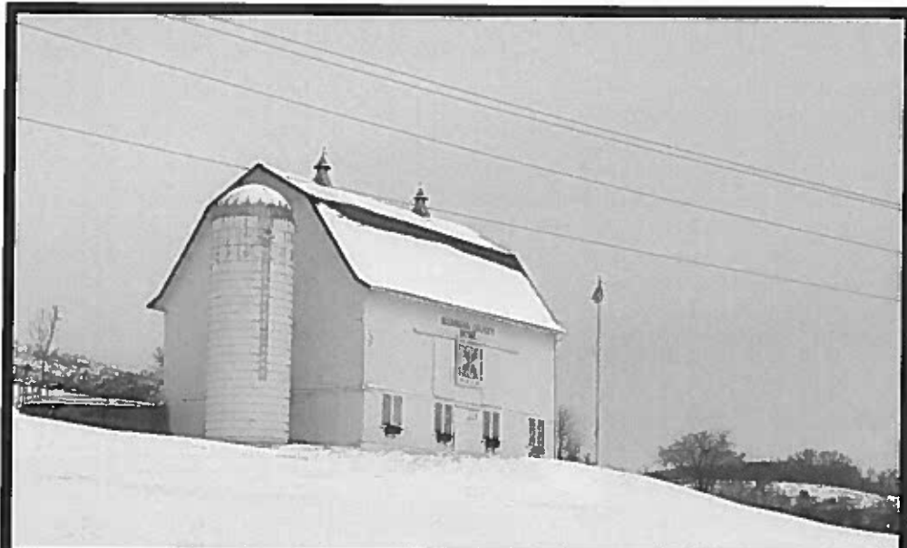
Photo #3.) Barn sits on Harrison County Home property as viewed from US 250 looking east from the County Home. Pumping station site and pipeline route is visible from this vantage point.
