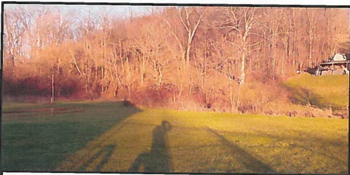
Photo #12) View from Northeastern corner of water treatment plant
