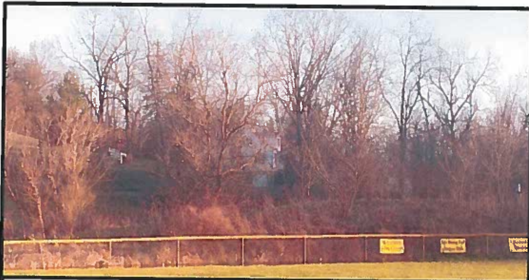
Photo #10) Looking east from corner of water treatment plant. There is a residential home mostly obscured by trees. Construction of the home appears to be modern.
