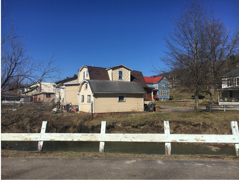
Historic Structure on South Side of East Main Street just west of Conotton Creek
